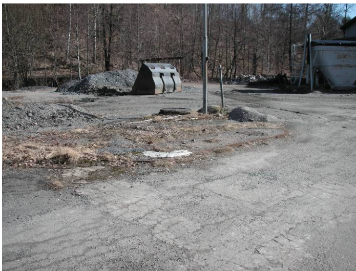
Betongplatta fd pump
